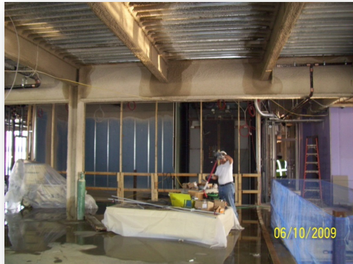
Figure A.4 Temporary Elevator Shaft Separation
