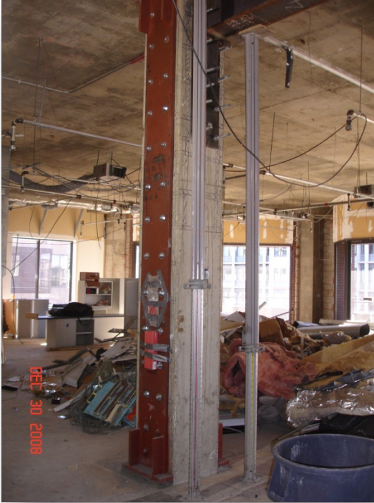
Figure B.2 Column Reinforcing
