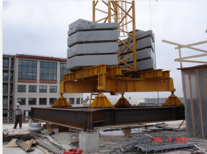
Figure A.6 Tower Crane Base and Cribbage
