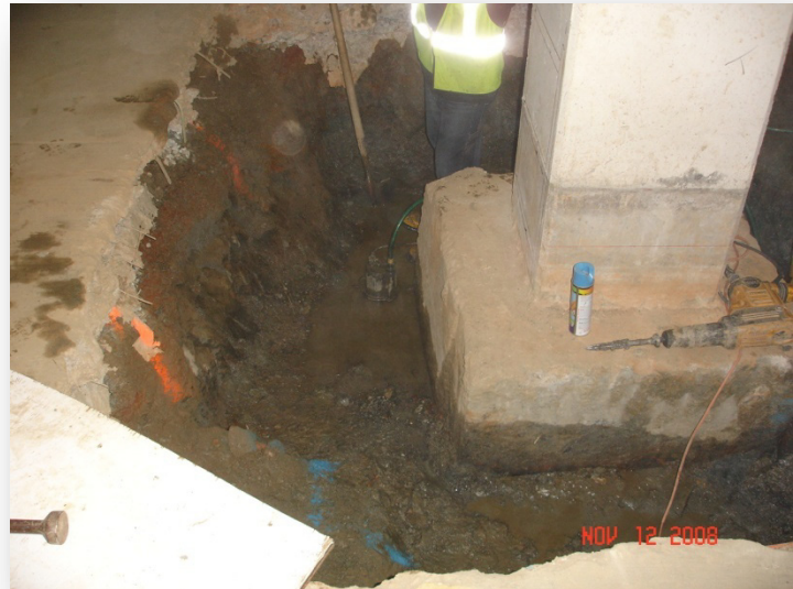
Figure B.1 Foundation Spread Footing Expansion
